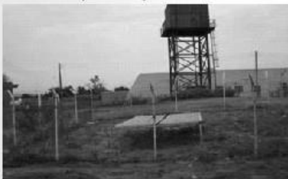
Solar Water Pumping for Students in Sokoto, Sokoto State
