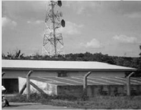
Solar PV for Telecommunication 20km Kaduna-Abuja Road
