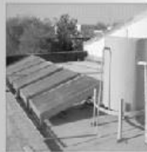
700L Community Based Pilot Water Heater Location: UDUTH Collector: 1000 litres Cost: ₦80,000.00 Year: 2008 Objective: Water heating Sponsor: SERC Beneficiary: Green Lancers World UDUTH
